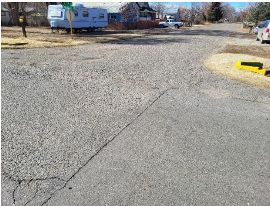
7 Transition between 2 pavement conditions
