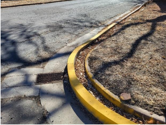
5 Existing inlet- drainage modifications may be necessary at some locations.
