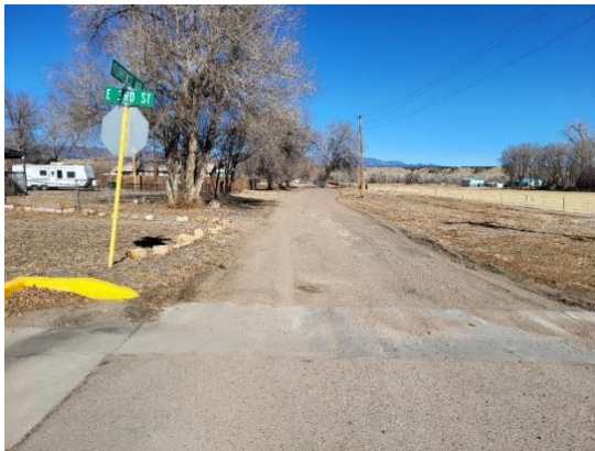
2 Unpaved Road- Florence Ave at 3rd St
